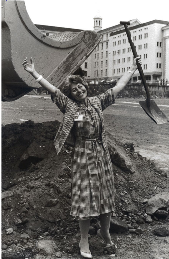
“Dr H Reeve Sanders, Superintendent of Groote Schuur Hospital, lifts the first sod – with bulldozer and shovel – on site.” 179
